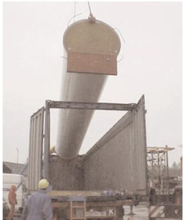
Loading antenna into container.
